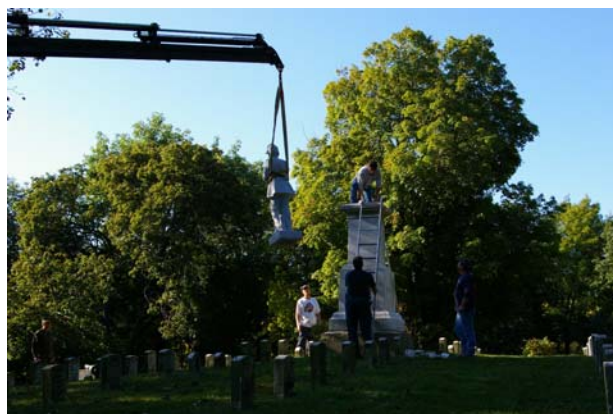
Hoisting the soldier into place.
